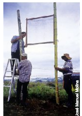
Construction of an SFC using bamboo posts in Columbia.
